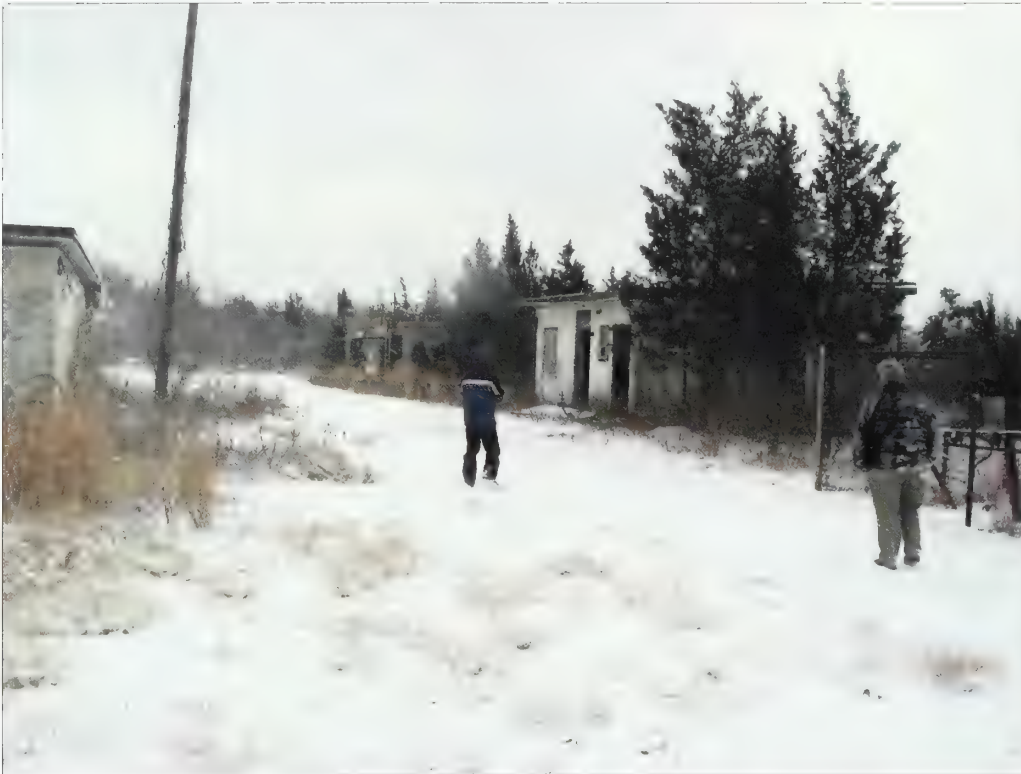
Figure 3.59. View looking southeast from vehicular route to Control Area #1, NIKE radar site. From each control area, a vehicular route leads to the Ready Barracks. From Control Area #1, the route is paved and ends in a hammerhead turnaround south of the Ready Barracks (Olmsted Center, January 2009).
